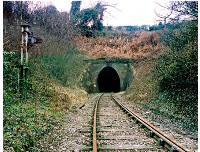
The west portal of Grove Tunnel in March 1986. Photo Nick Catford
